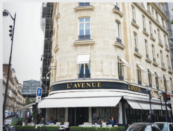
41 AVENUE MONTAIGNE 75008 PARIS
